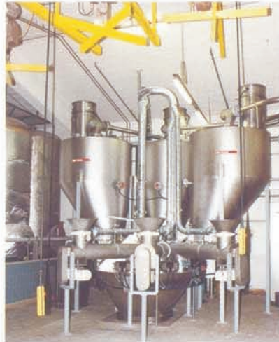
Ingredient-feeding for detergent production with weigh vessel and receiving stations for FIBC big bag discharge
