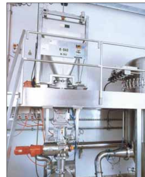
Reconditioning system in a pharmaceutical plant showing a container emptying station, a prebraker nibbler, a rotary valve and a mill before powder is conveyed into an explosion-resistant receiving vessel and downstream to a tablet press.
