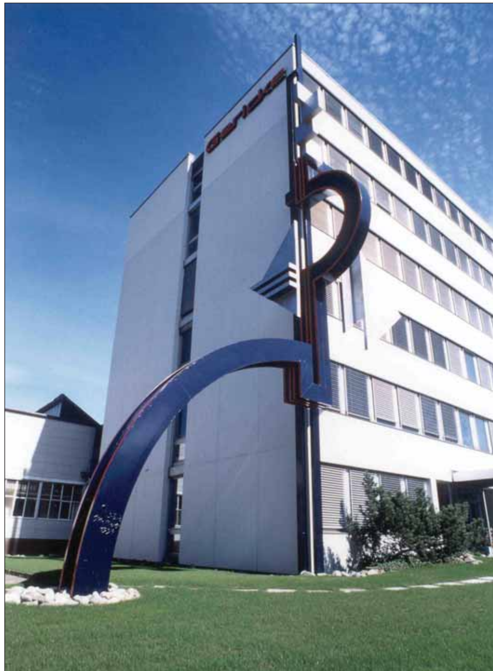
Gericke head office in Regensdorf, Switzerland.
